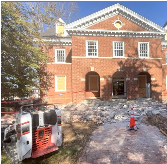
Exterior Concrete Demolition
