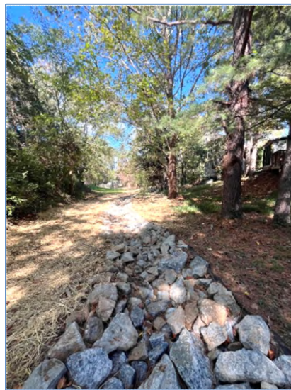
Repaired Channel (After)
